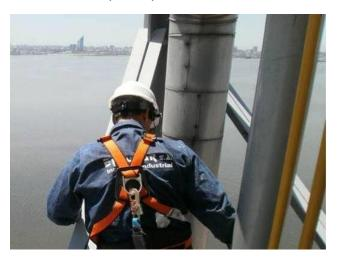
In 2011, the 78m tall flare stack, located in the Bay of Montevideo, previously hot-dipped but depleted, was protected with 2 layers of **ZINGA**.
