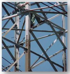
System: Surface preparation: Manual steel brush, sand-paper, degreasing ZINGA 2 x 40 µm DFT
