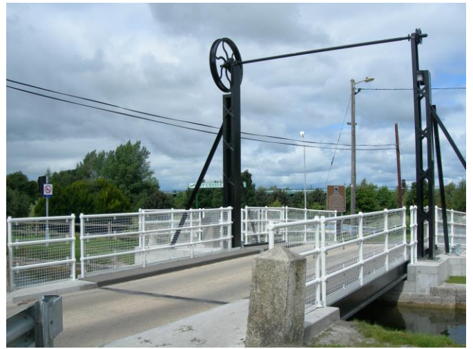
A closer view of the surface of the deck
