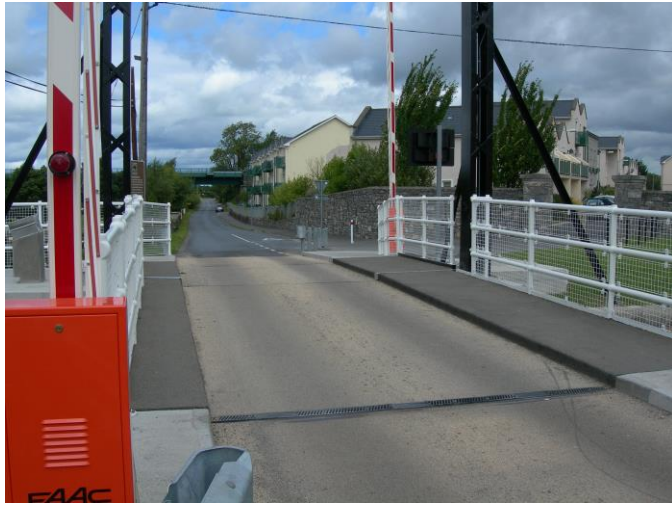
A view of the bridge approach
