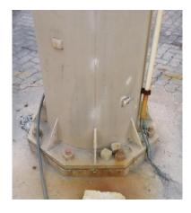
The 45m high lighting poles, originally hot dip galvanized, began to show signs of corrosion after more than 20 years of service.
