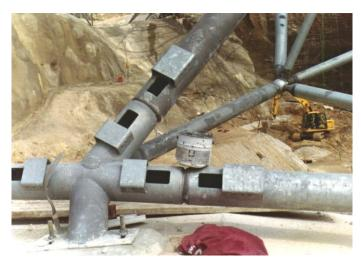
For aesthetic reasons, **ZINGA** was overcoated with a vinyl aluminium paint. **ZINGA** was used to repair the HDG layer (damaged during transport and assembling).
