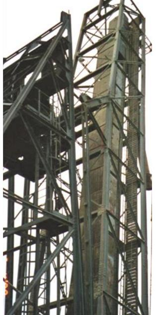
These two cranes and the conveyors were heavily corroded and it has been decided that they had to be protected by an anti-corrosion system providing cathodic protection: **ZINGA** was chosen.
