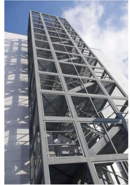
The fire escape staircase was originally hot-dipped and has been reloaded with ZINGA to give it renewed galvanic corrosion protection.
