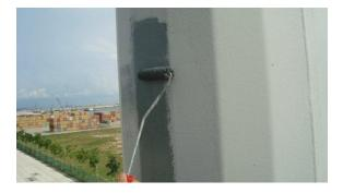
More lighting masts are being protected with **ZINGA** to recharge the 15-year-old, worn out, hot-dip galvanisation.
