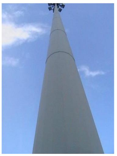
System: Surface preparation (on old hot-dip): Wire brushing and wash down ZINGA 2 x 60 μm or 2 x 80 μm DFT
