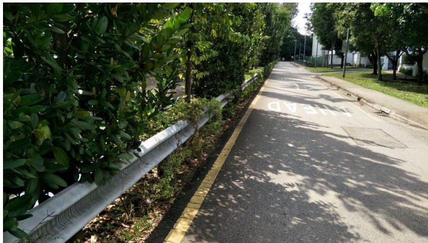
Condition survey of KAMPONG JAVA Road Rails in December 2017, 13 years after ZINGA application.
