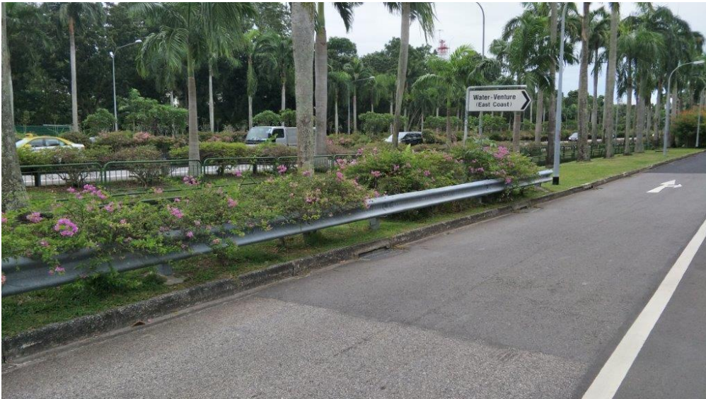
Condition survey of ECP SERVICE Road Rails in December 2017, 13 years after ZINGA application.
