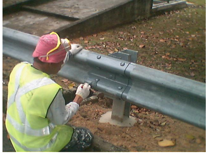
Condition survey of ECP SERVICE Road Rails in December 2017, 13 years after ZINGA application.
