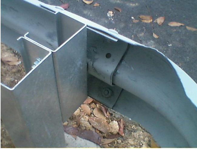
Condition survey of ECP SERVICE Road Rails in December 2017, 13 years after ZINGA application.
