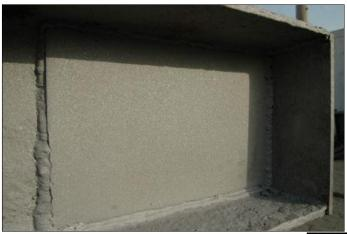
System: Surface preparation: Sand blasting SA 2,5 Application in duplex system: ZINGA 2 x 60 µm (brush)
