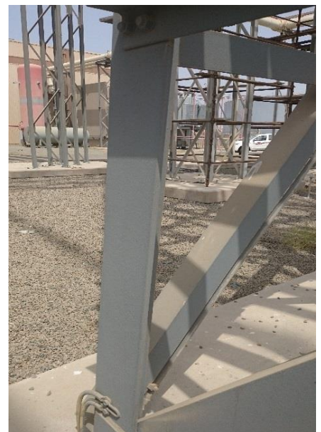
Final result 1 year after application
