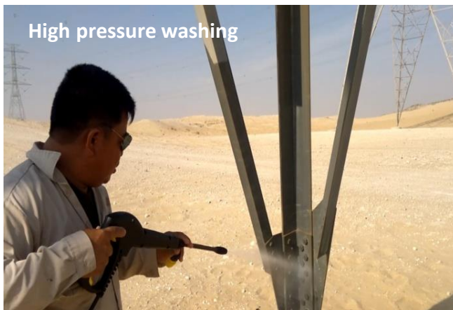
Pylons prior to ZINGA treatment
