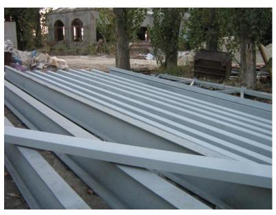
System: Surface preparation: Blasting SA 2,5 and Rz 50-70  $\mu$ m ZINGA 1 x 80  $\mu$ m DFT
