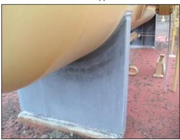
System: decontamination by UHP cleaning blasting to SA 2,5. Zinga 2 x 90 µm DFT
