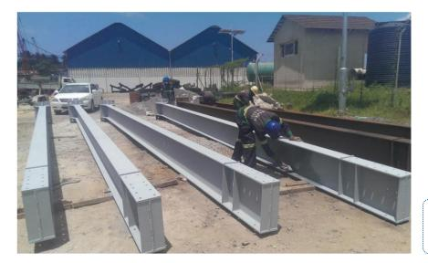
In 2015, the structural steel beams of the KPA Dockyard were treated with **ZINGA** to protect them from corrosion in the harsh marine environment.
