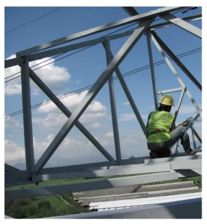
In May 2011 a first high tension pylon (150kV) was protected with **ZINGA** because textile industries had severely attacked the old hot-dip.
