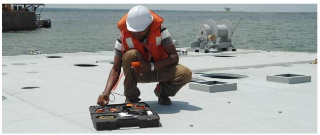
In 2012, a 200m² barge was protected with a three-coat system based on **ZINGA**. This system will provide an active protection and an anti-skid surface.
