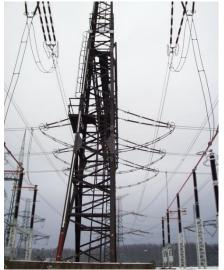
On some joints **ZINGA** is covered by the Czech paints HS-Elastcom or Rezdico. These paints were not intended as a protection but were used to obtain a similar colour as Atmofix.
