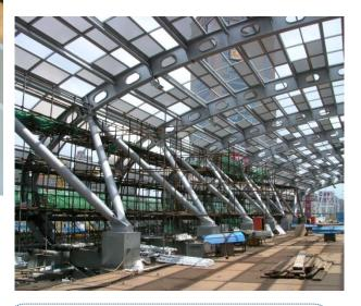
System:ZINGA1 x 50 μm DFTEpoxy MIO1 x 100 μm DFTPU1 x 60 μm DFT
