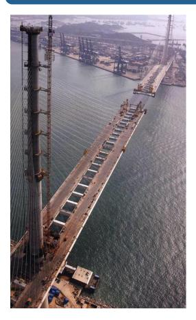
The Stonecutters Bridge is a high-level cable-stayed bridge which spans the Rambler Channel in Hong Kong, connecting Nam Wan Kok, Tsing Yi island and Stonecutters Island. The bridge deck was completed on 7 April 2009, making this the 2<sup>nd</sup> longest cable-stayed span in the world at the time of its completion. It opened to traffic on 20 December 2009. The bridge spans 1.6 km, with 3 lanes in each direction.
