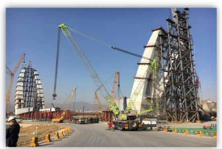
Coating with **ZINGA** started in 2017. In total **182 tons of ZINGA** was used (internal and external of steel structure).
