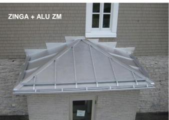
System:Surface preparation :SSPC SP-1/SP-7ZINGA (areas without visible corrosion):2 x 40 μm DFTZINGA (areas with visible corrosion):1 x 120 μm DFTALU ZM:2 x 40 μm DFT
