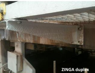
After 24 months, the **ZINGA** system showed no signs of corrosion. All supports not treated with **ZINGA** received the **ZINGA** system after 18 months
