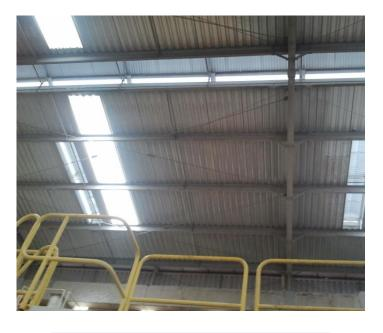
Roof over the wet end of paper machine #4 was totally rebuilt in 2008 using HDG carbon steel structure. In December 2010, the renewed roof using galvanized structure (only after 2 years) showed signs of oxidation.
