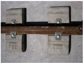
The railway company **DORBRAS** was looking for a solution for the oxidation on the metal plates that are used for the fixation of rails onto the crossbeams. In April 1999 approx. 45,000 Zinganised fixation plates were installed. A layer of 80  $\mu$ m **ZINGA** was applied with a spraying gun. These plates are constantly in contact with the concrete block at the end of each crossbeam and are slightly shaken each time a train passes on the tracks.
