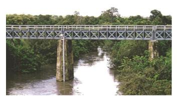
System: Gritblasting to SA 2.5 ZINGA 2 x 60 μm DFT
