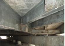
These pictures clearly indicate the high degree of corrosion before refurbishment with the ZINGA system.
