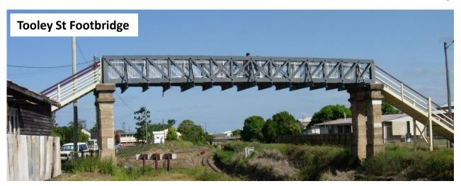
The below Queensland Rail Bridge was protected with **ZINGA** on 26-06-2003. The bridge identification number 902-788 was coated according to **Queensland Rails specification**. On June 20, 2007, an inspection was performed.
