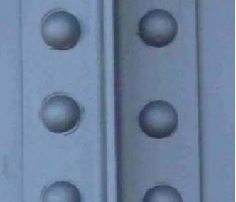
Typical view of **ZINGA** coated steelwork. All rivets, edges and bolts were stripe coated.
