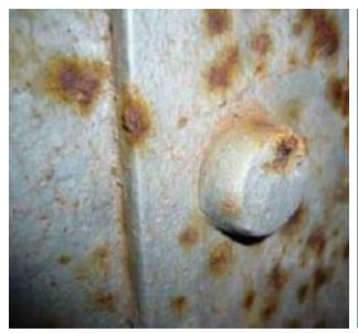
Site inspection in May 2007. (before **ZINGA** application) Note the increased beam corrosion.
