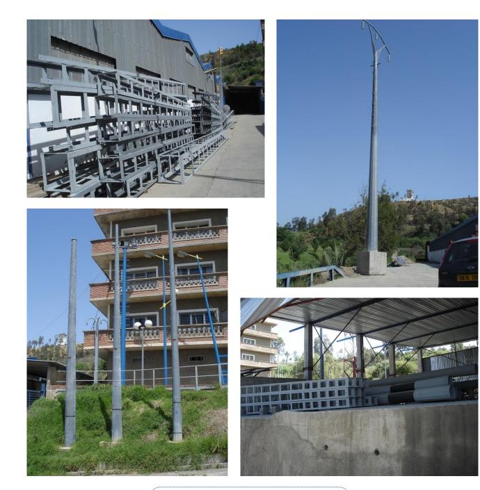
System: ZINGA 2 x 60 µm DFT on new steel
