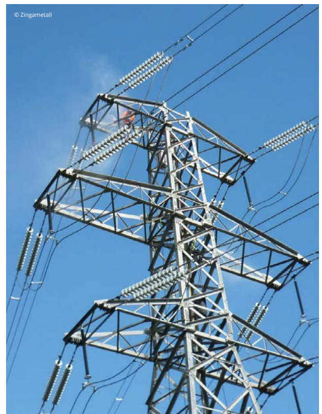
Figure 2 - Vapour-blasting an electricity pylon.
