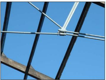
Above: The roof beams are all made from timber, and the steel tie-rods were zinganised.
