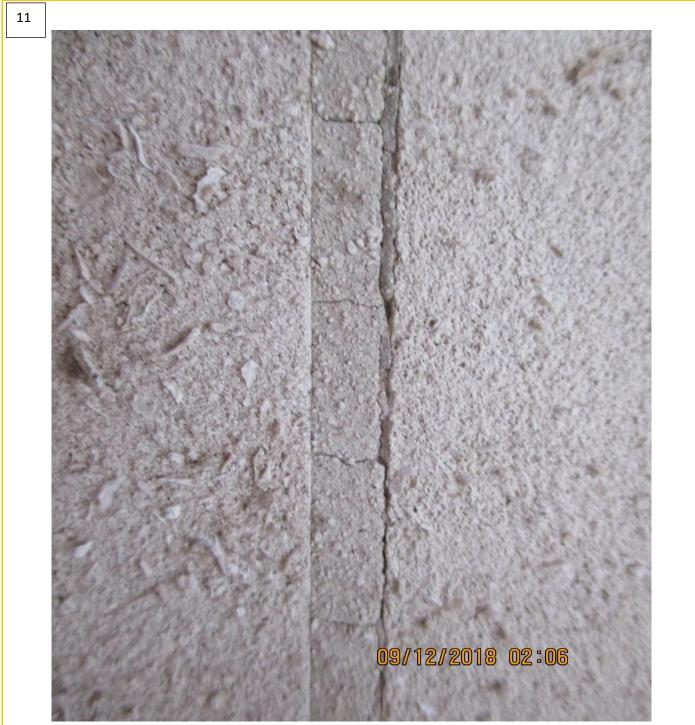
The previous pointing on the steelwork is not compatible and is breaking up. This could potentially allow the ingress of water/water-vapour that can have a long-term effect on the steel beams.
