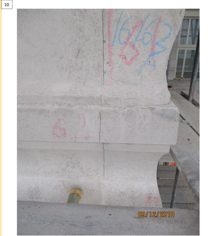
Another area where the expansion of corrosion products on the beam is putting pressure on both the inner cementitious layer and the outer stonework. This is no different to the spalling seen on reinforced concrete.
