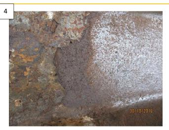
Massive volume-expansion of corrosion products
