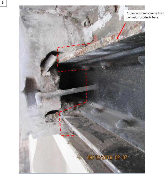
Exposed beam and 'T' tie-bar. The dotted lines show the air-gap being built in when closing up. The new cement will have a gap of 25 mm between the steel and cement to allow for volume expansion of corrosion products over the next 100 years or so.
