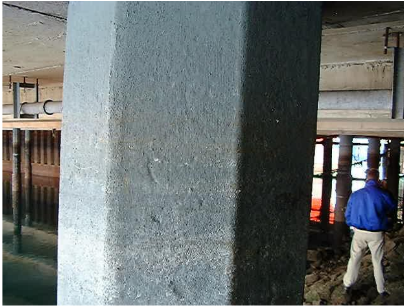
August 2001 : Zinga was applied at 4 x 50 \mu m DFT between high tides. This project was insured and inspections done by SGS in Brugge
