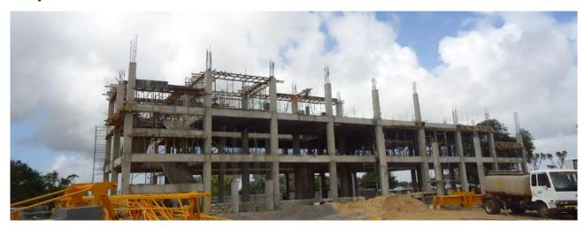
At this point, about 3T ZINGA has been applied in 40µm DFT on 350T of rebars.
