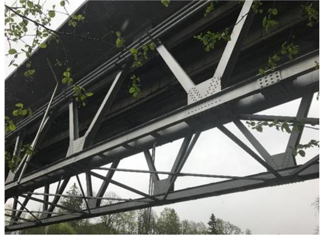
These photos are from **May 2017, after 15 years of exposure**. The system is still intact without any sign of breakdown or failures. Even in complicated areas such as around bolts, nuts and rivets there are no failures. The system is believed to protect the steel structure for many more years to come.
