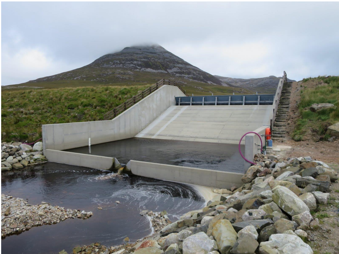
Two views showing the concrete spillway as viewed from the bottom end
