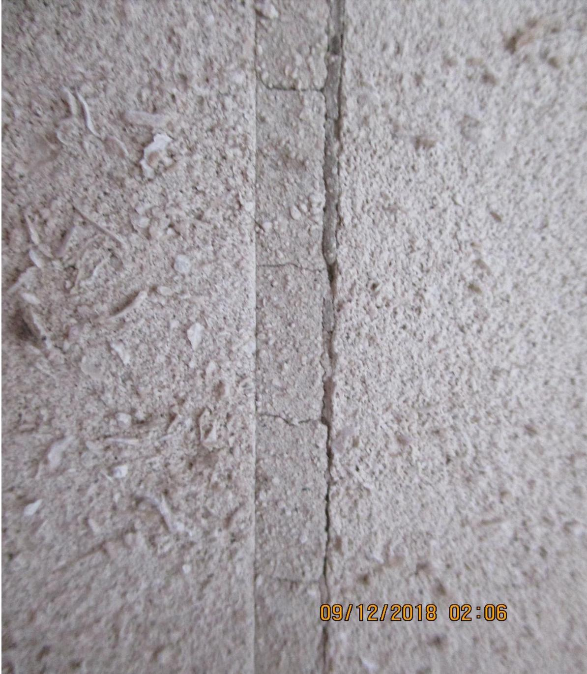
The previous pointing on the steelwork is not compatible and is breaking up. This could potentially allow the ingress of water/water-vapour that can have a long-term effect on the steel beams.
