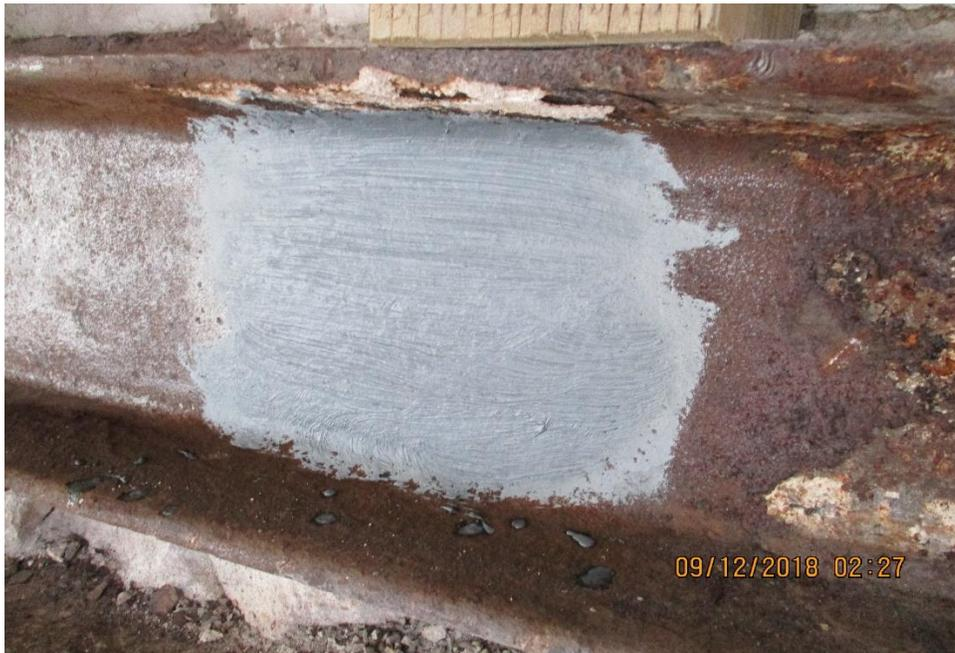
The first test-section is coated so that the application quality can be evaluated and the drying-times observed.
