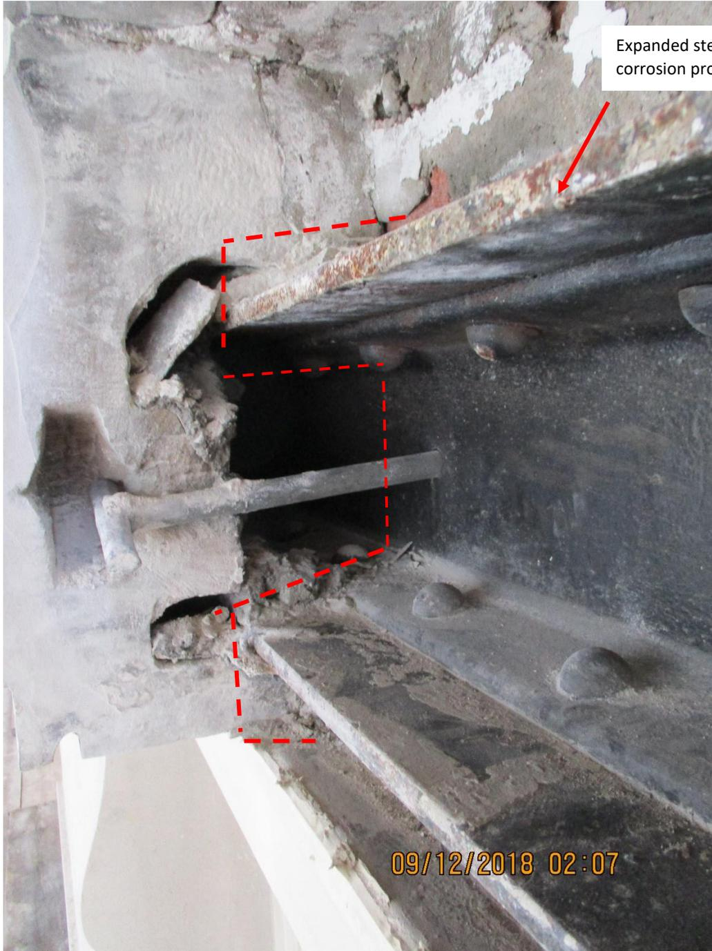
Expanded steel volume from corrosion products here
