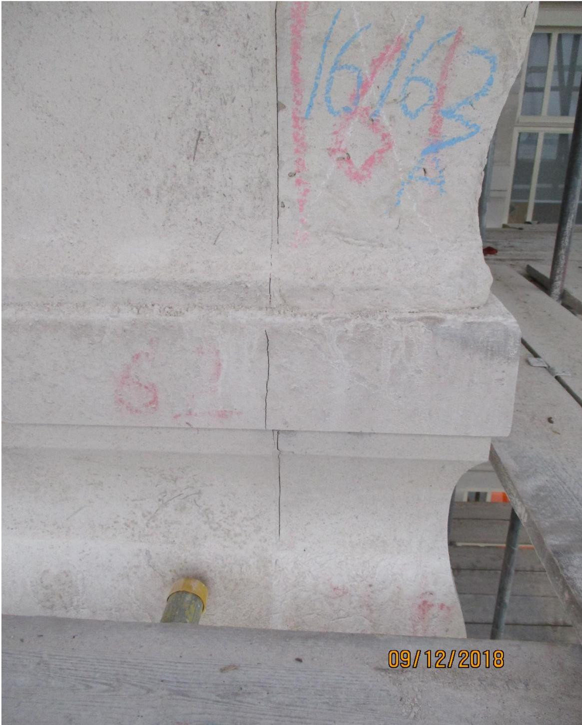
Another area where the expansion of corrosion products on the beam is putting pressure on both the inner cementitious layer and the outer stonework. This is no different to the spalling seen on reinforced concrete.
