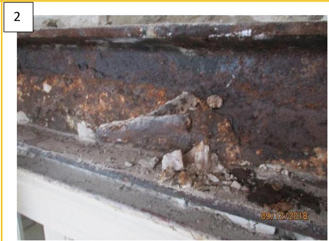
Heavy corrosion is prevalent along north east wall
