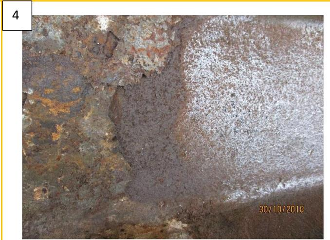
Massive volume-expansion of corrosion products
