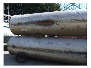
To protect the **London Eye** from the busy boat traffic on the Thames there are 10 barrage pontoons placed on both sides of the wheel. The coating on these pontoons were in a quite bad state and needed to be refurbished. In November 2014 the **ZINGA Distributor** in the U.K., **MGDUFF International** received the order to apply 2 **ZINGA** systems on the 10 pontoons.
