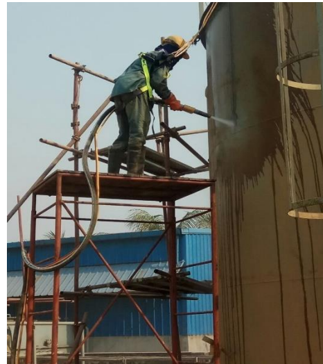
Vapour-blasting with a Satblast unit
