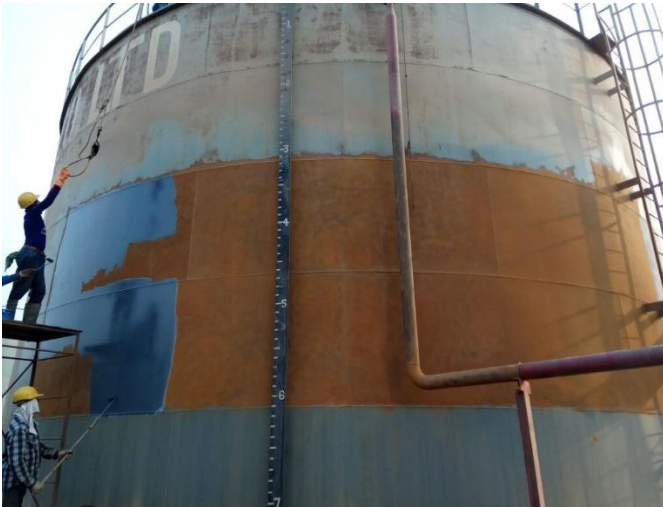
Removing the old coating system
