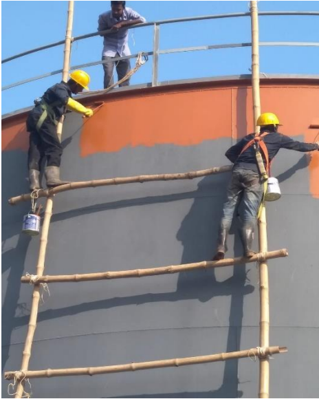
Home-made scaffolding – PU application
