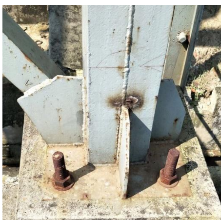
Condition before surface preparation & application of ZINGA
