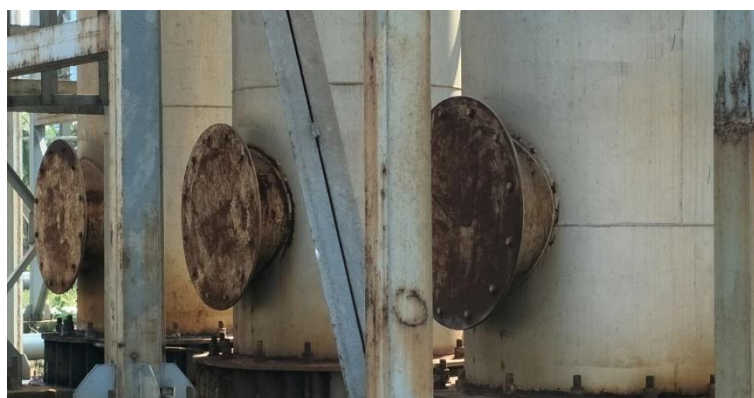
Condition before surface preparation & application of ZINGA
