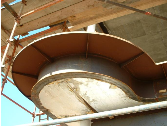
The steelwork above the curved glass in the living room
