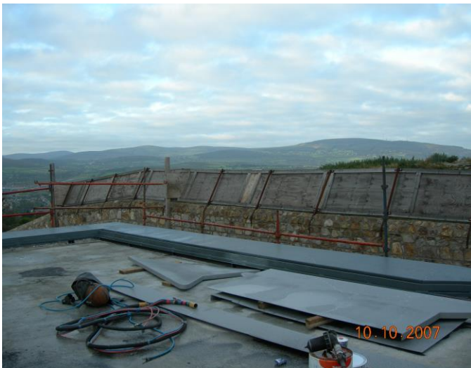
Another section-view of the large roof area
