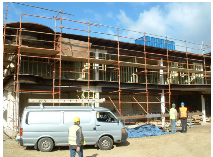
A view showing the lateral H-beams that were hidden by brickwork
