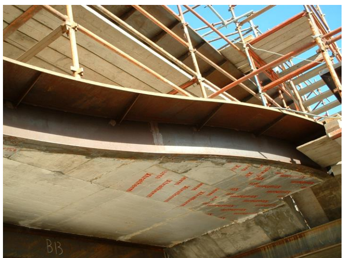
The massive steel canopy over the front door of the house
