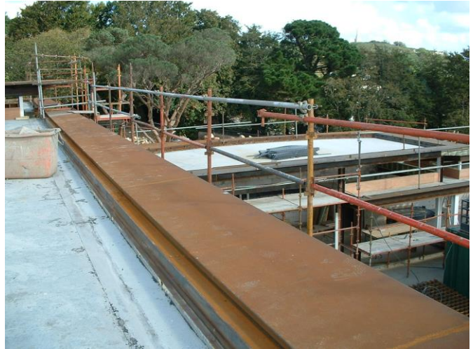
The steel edging-panels around the entire roof
