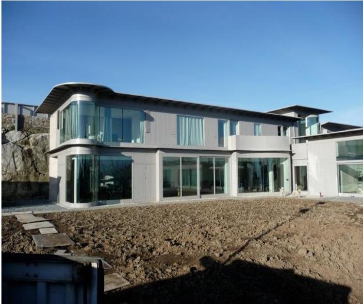
Front view of the house after completion showing the steel canopy
