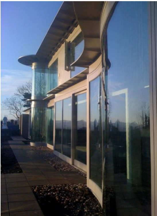
A side view showing the amount of steel used
