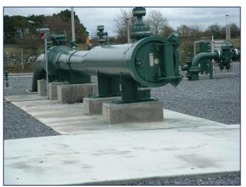
This pumping station pumps gas from the Corrib Field onto the shore in Galway. The manifolds and other assorted pipe-work were delivered to site as new, uncoated steelwork and due to the proximity of the sea it was decided to galvanise all of the steel with Zinga.
