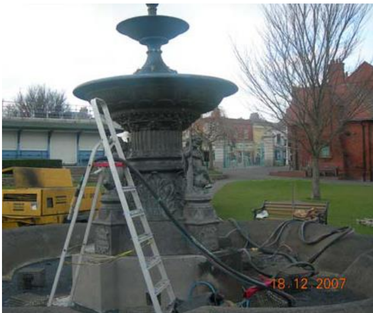
Blast cleaning to remove the old paint. (picture taken on 18-12-2007)
