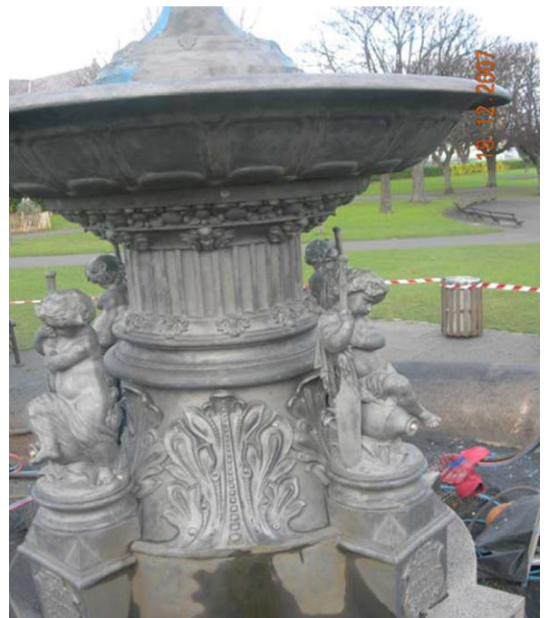
Detail of the fully blasted fountain
